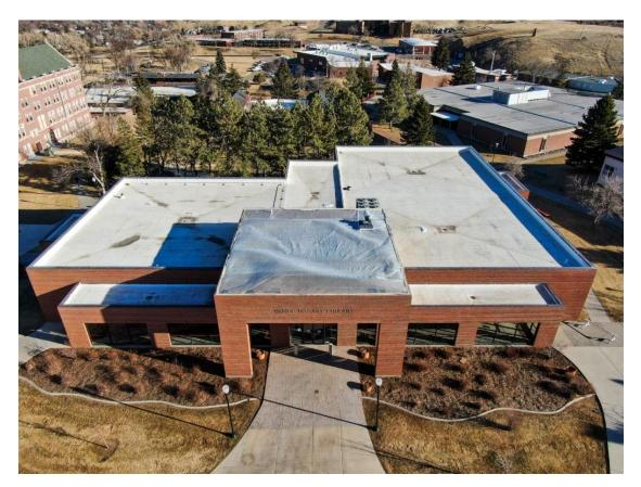
MSU-Northern's Vande Bogart Library roof was damaged on Wednesday (Jan. 13) due to the high winds. The main entryway roof was damaged in three areas, mainly over the mechanical equipment loft. No one was hurt when the waterproof membrane and some perimeter framing blew off due to extreme wind gusts.
