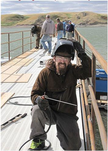
MSU-Northern's welding professors and students welded a handrail on the Handicap fishing dock at the first lake. This is a much needed addition to the lake and will make it safer for everyone.
